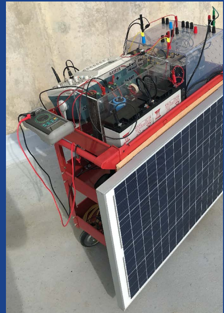
Capt Lorio's research included a DC microgrid set up with a PV array, step-down switching DC-DC converter, lead acid batteries as the energy storage system and load, and an Opal-RT real-time simulator for rapid control prototyping.
