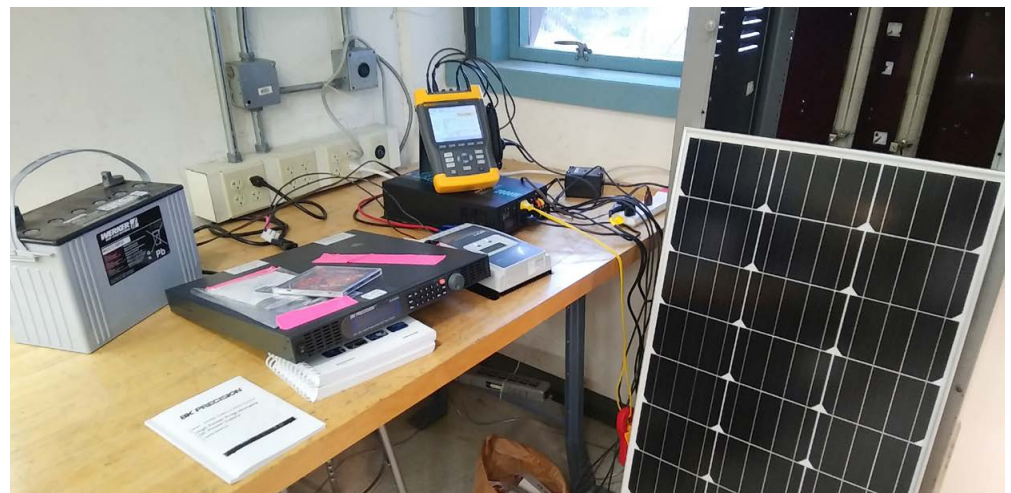
Hastily-Formed Microgrid project (HFM) utilizes commercial-off-shelf (COTS) components.
