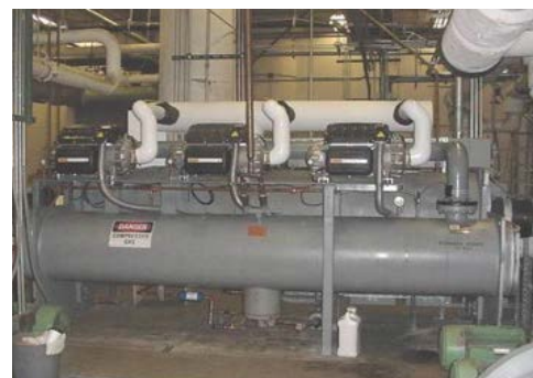
Magnetic Bearing Chiller at Naval Base San Diego (Source: Kistler, Paul. Transition of Magnetic Bearing Chiller Compressor to Navy-Wide Use. Presentation to Tri-Service Facility Technology Transition Collaboration Meeting. March 2011.)
