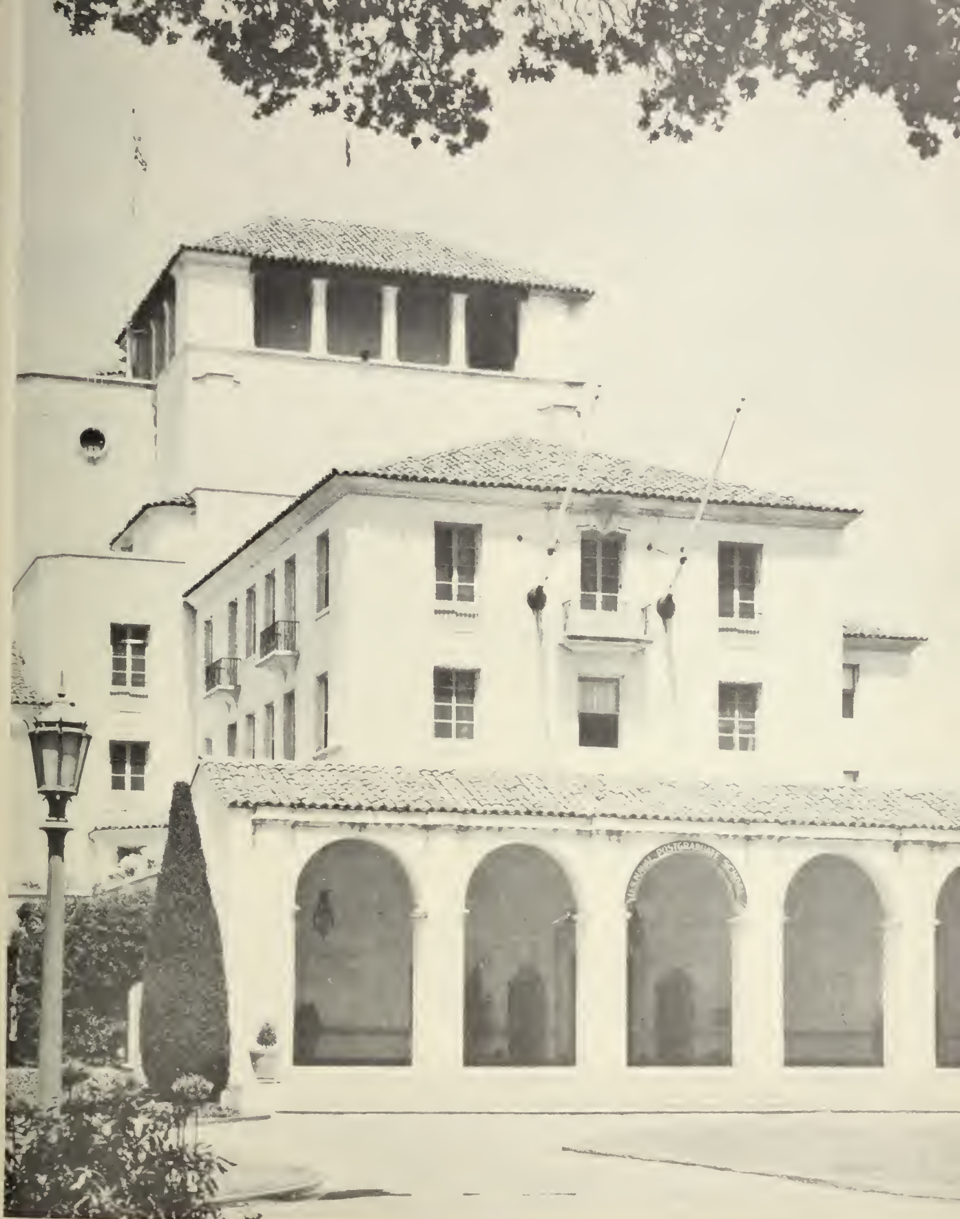
Entrance to the Main Building, which houses the Administrative Offices and Bachelor Officers' Quarters of the U. S. Naval Postgraduate School.
