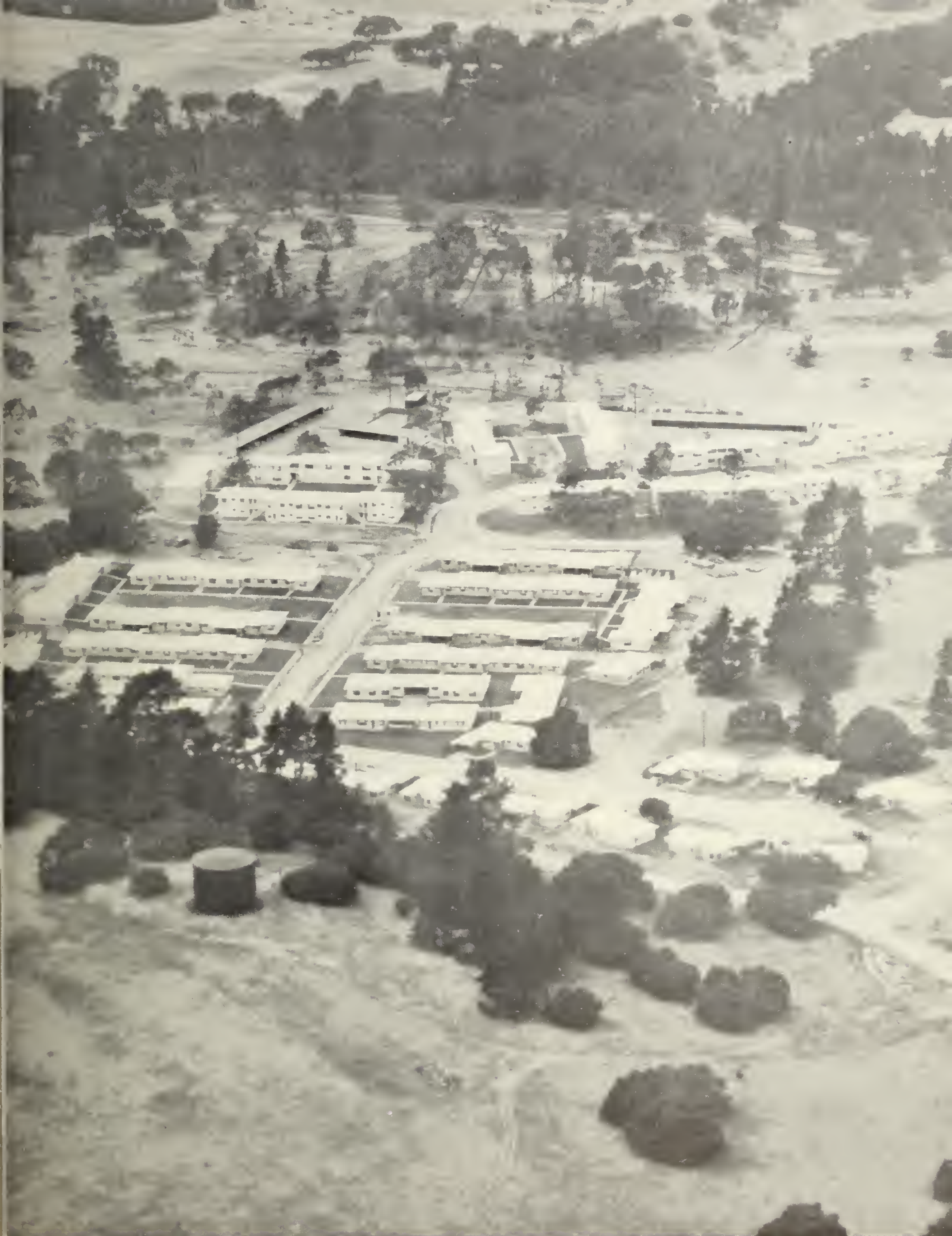
Aerial view of "La Mesa Village," Wherry Housing Project.
